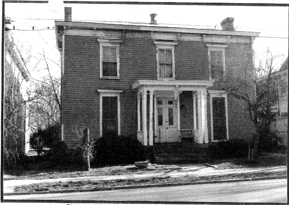
Plate 1. West Washington Street (123-096-0141). One of the more stylish houses on West Washington Street.
