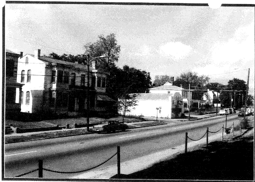
Plate 5. Double House (123-096-0134) on corner of West Washington Street and Jones Street.
